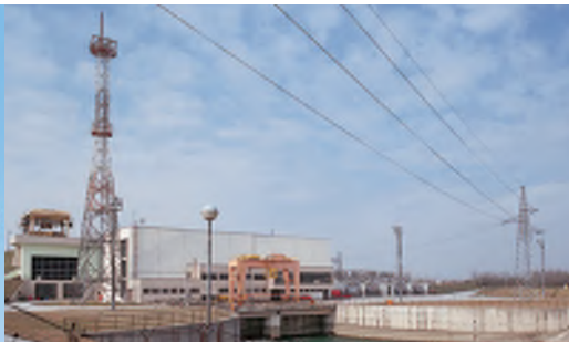
Dubrava HPP antenna mast
