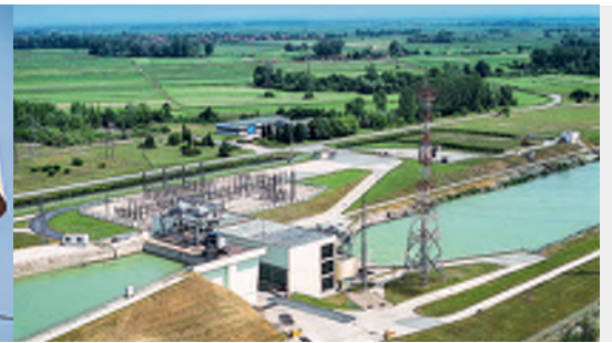
Čakovec HPP antenna mast
